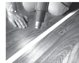
Heat the seam area.
