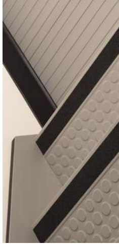
Tactile Warning Surface shown above.
